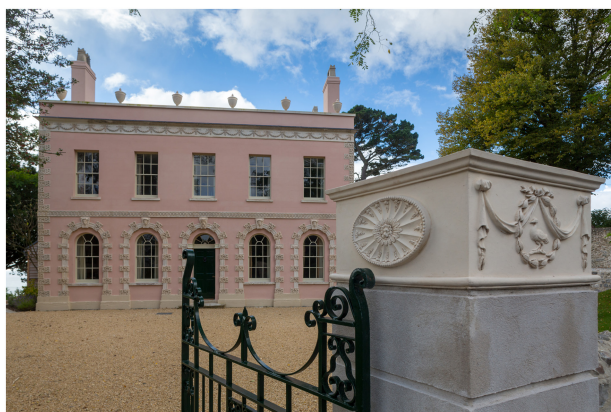
FIGURE 4 An 18th-century Coade stone gate cap from Eleanor Coade's own seaside villa at Belmont in Lyme Regis, Dorset, which she acquired in 1784 (photo: Caroline Stanford)
