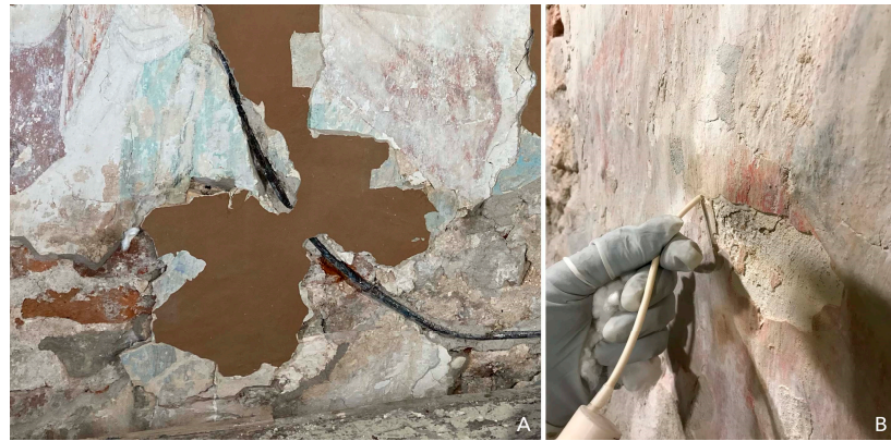
Figure 11. Chapel's fresco during the restoration works. (A) Restoration process in the opening up of the fresco (photo: M. Rasiņa, 2020); (B) conservation process by the introduction of lime-based injections (photo: M. Rasiņa, 2021).
