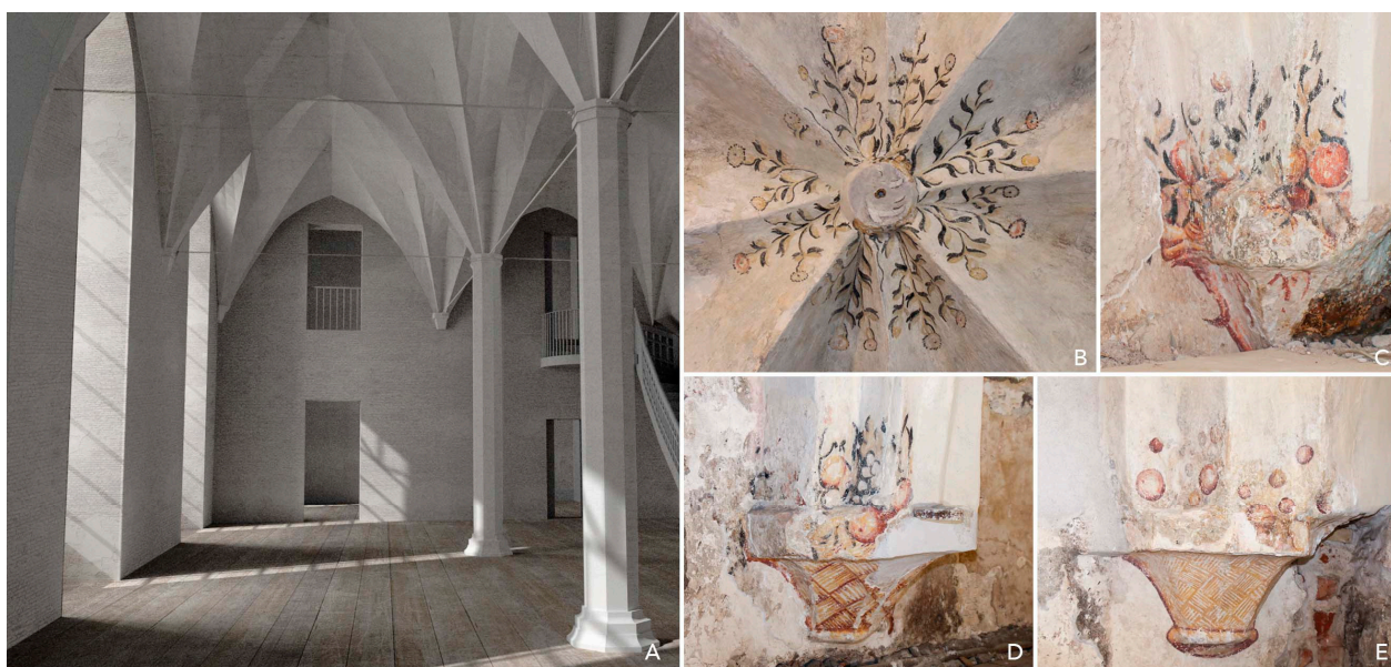
Figure 4. Refectory of the Riga Castle. (A) 3D visualisation of the possible look of the premise after restoration by architect Reinis Liepiņš, 2015 [1]; (B) vaulting's central painting after opening and restoration (photo: M. Rasiņa, 2020); (C–E) consoles after restoration (photo: M. Rasiņa, 2020).
