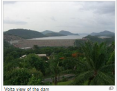
Volta view of the dam
